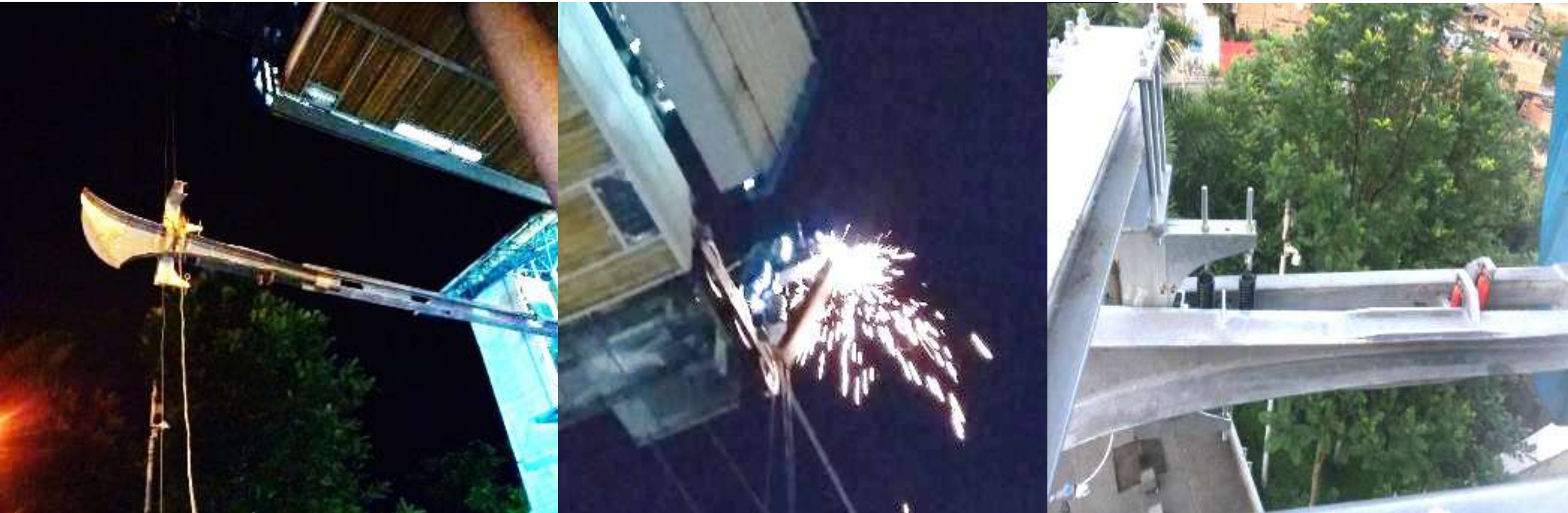
Change of stabilization rails in stations
