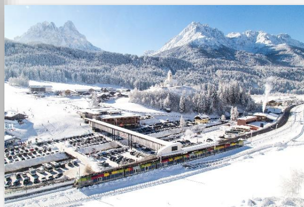
Figure 6 - railroad connection 3 Zinnen Dolomites
