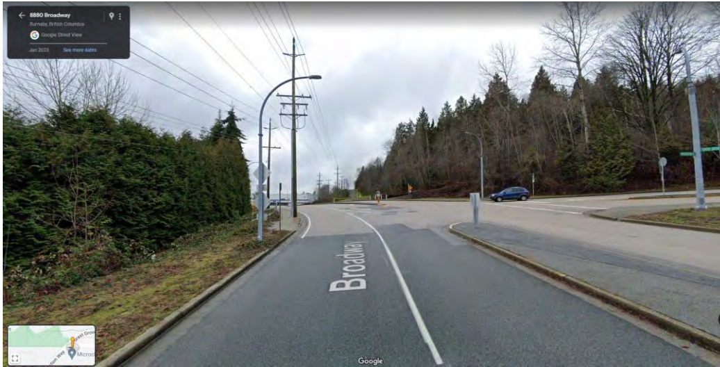
BC Hydro 69kV Transmission w/ Distribution
